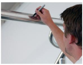
Using the pre-drilled holes in the top section tube, mark the drilling positions on the front leg tubes.
